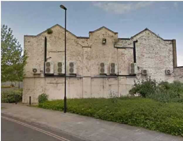
Image: The southern gable wall of the existing building
